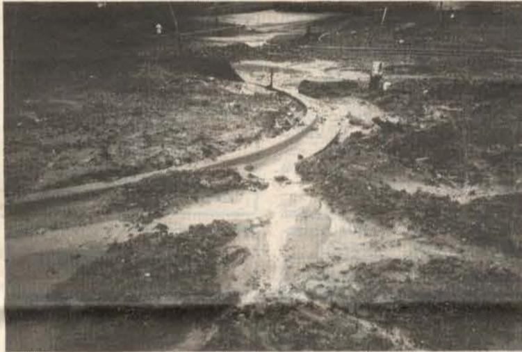
"On Saturday a torrent of water washed out sections of two earth berms constructed to channel run-off to a makeshift pond at the head of St. James Place." The above photo shows the route the water took along the new curb toward St. James Place. — photo by Jim Sterling
