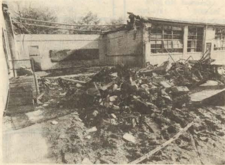
The St. Hugh's School fire left a room on the west side just behind the auditorium completely devoid of its outside wall, roof and contents. — photo by J Henson
