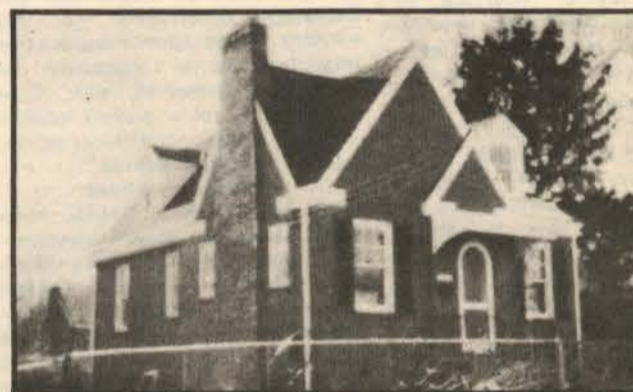
SILVER SPRING — TWO FIREPLACES, GARAGE are only 2 fine features in this solid brick 2-story home. Also separate dining room, remodeled kitchen, full basement and huge expandable 2nd floor. Buy this home with only 5% down payment. $73,500. Call now, 345-2151.
