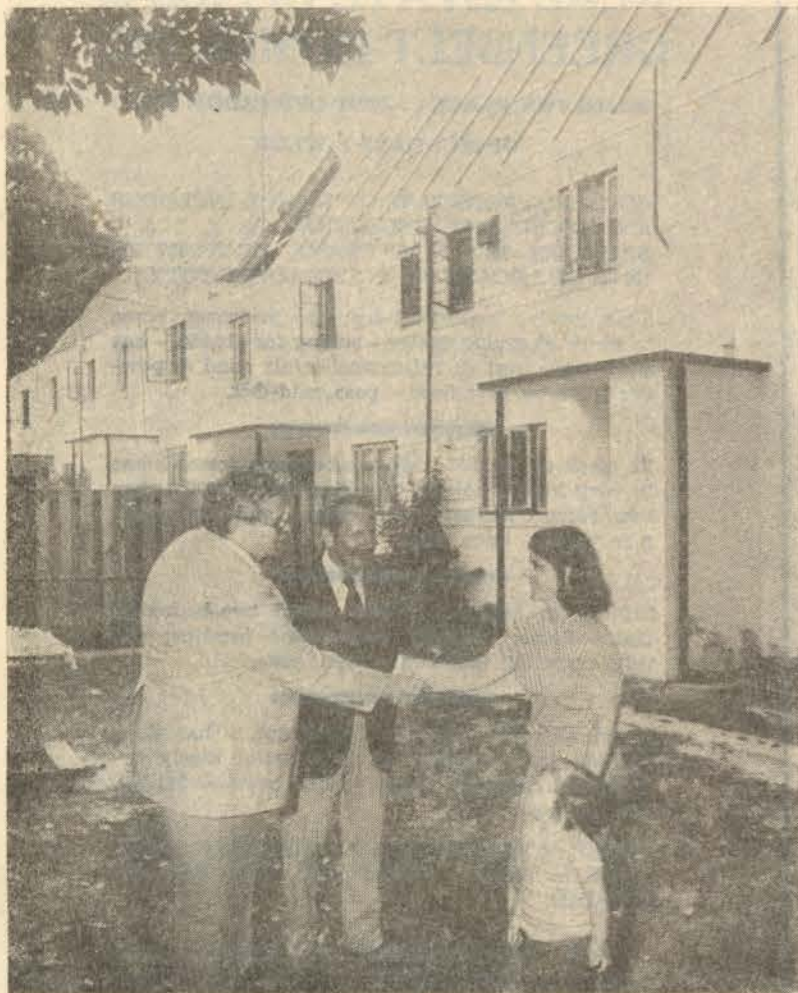
Under a backdrop of solar panels, the muscle of the Greenbelt Homes, Inc./Goddard Solar Energy Research Project, Royal Breashears, general manager of GHI talks with Mrs. Kathy Rellihan, member-owner of one of the four units served by the project. Emil Hymowitz, Project Manager looks on. — N.A.S.A. photo
