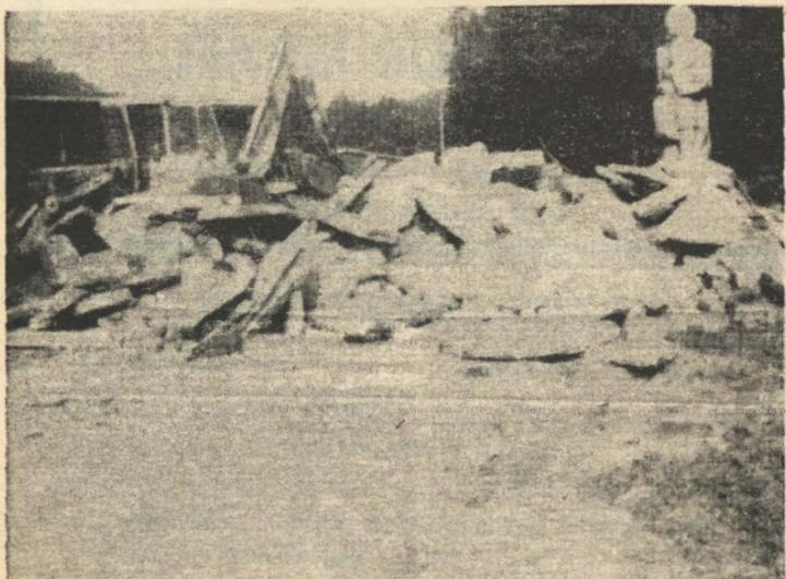
Back hoe - bulldozer doing its thing tearing out old cement walkways in the Center Mall. Refurbishing will include new brick-like bomanite walkways and more plantings. See story.
